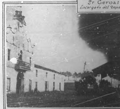
Vista exterior del Barracón
